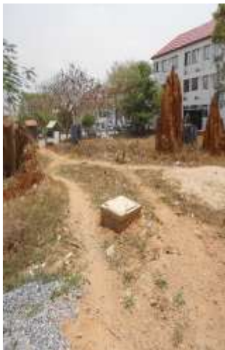
Sewage Line Chamber Presence
