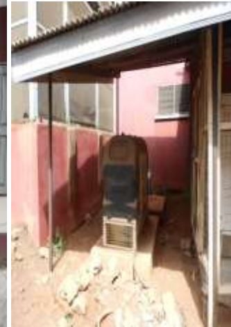
Relocation Generator Set 2
