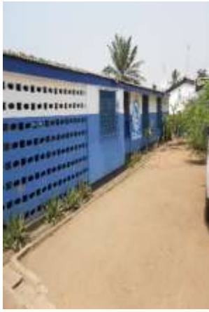
Frontage of GNA Office Building
