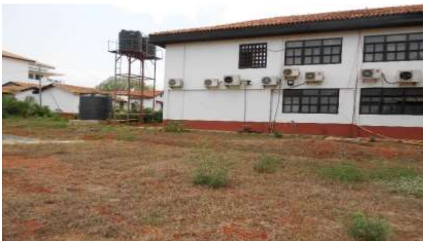
Back of the Existing Biotechnology Centre Building
