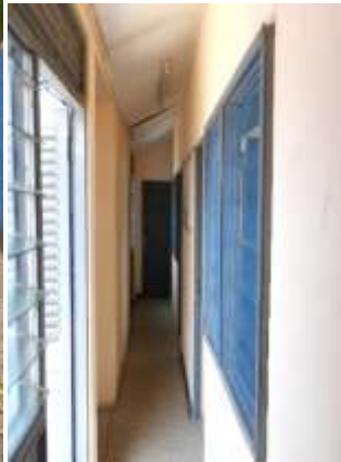
Interior Corridor Features
