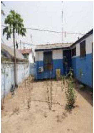
Back Section of Building
