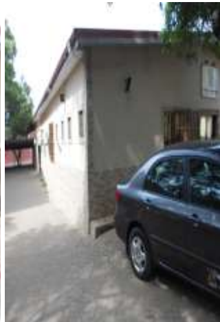
Partial Demolition (Animal Hse Bldg)
