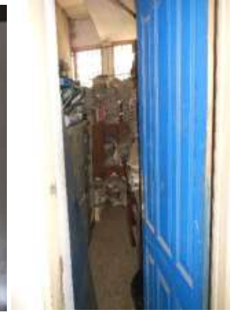
Old Storage Room
