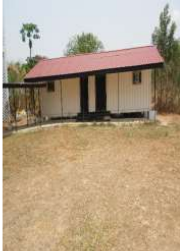
Relocation of Metal Container
